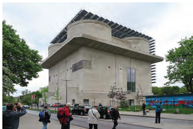
The massive and brutal outline of the Wilhelmsburg Flak Tower. The metal slats are solar panels and part of the recent refit. Mostly refaced, areas of the bunker's walls have been left in original condition
